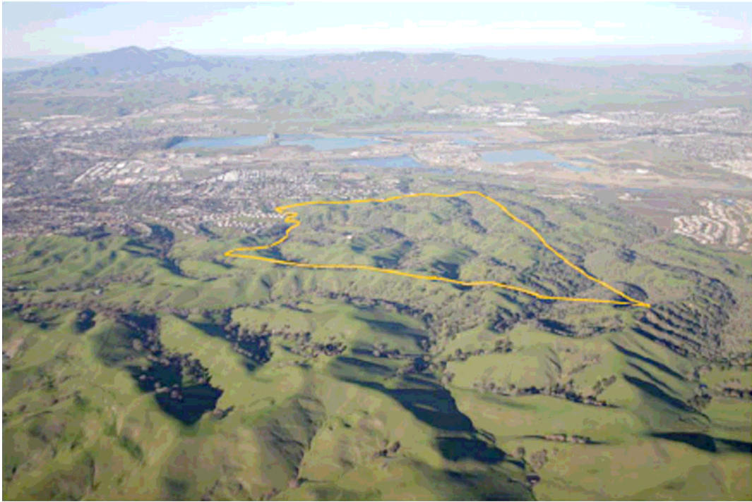
Figure 2: Aerial Photograph Looking to the North
